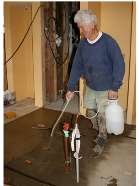
Preparing the layer below for more mud
