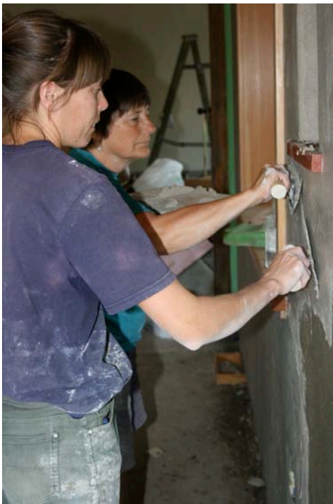
Cindy and Karen applying the final coat of plaster on the inside walls
