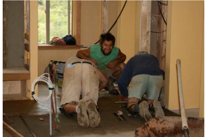
Mikey, Silas and Terry hamming it up with trowelling the final coat on the floor
