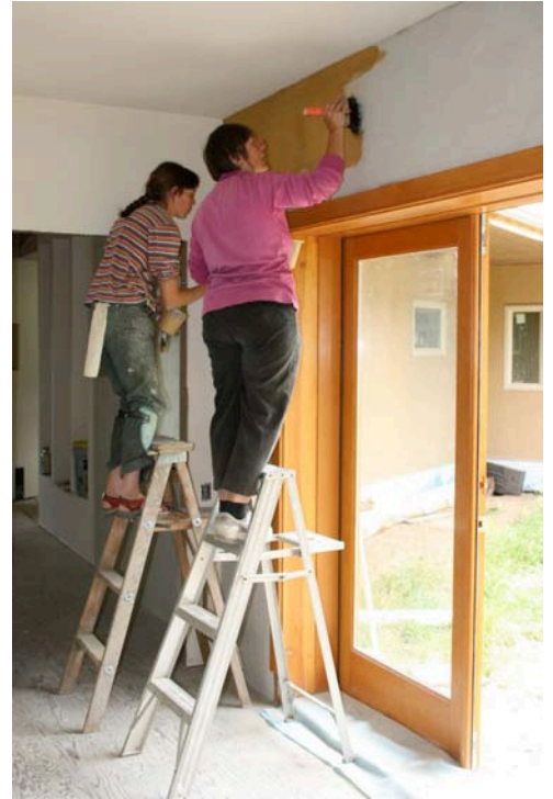
Colouring the walls with an ochre aliz
