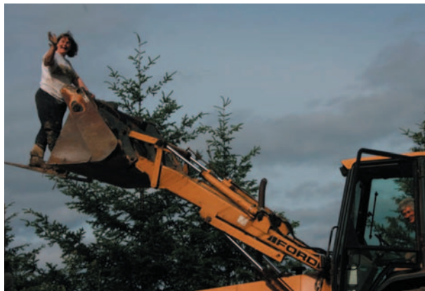
Teri getting a ride down from the top of the wall at the end of the day
