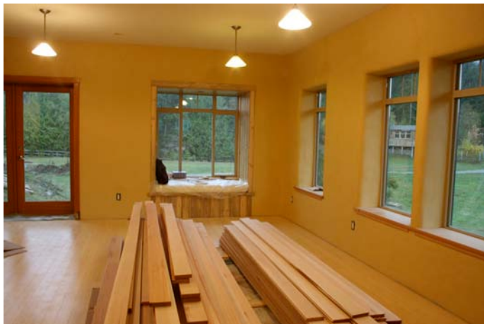
Studio with bamboo flooring installed. Douglas fir is stacked awaiting installation elsewhere in the house.
