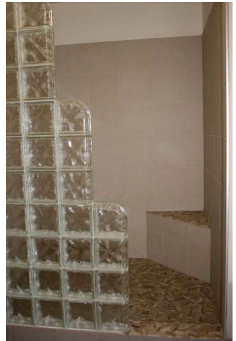
The floor and walls of the shower in the master bathroom are tiled and separated with a glass wall.
