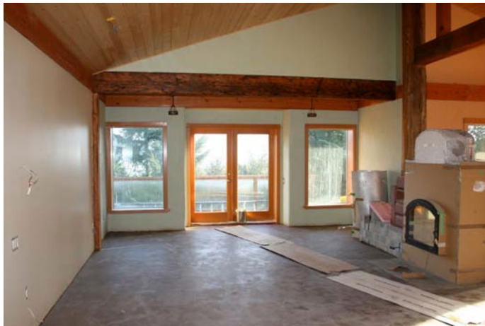
Earthen floor coated with beeswax/carnauba wax/earth pigment/thinner mix.
